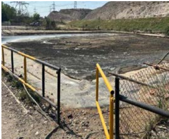
Figure 17: Leachate Collection Pond
