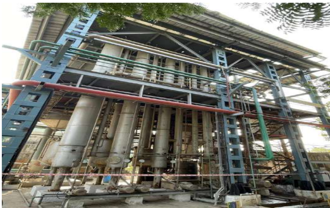
Figure 19: Multi-Effect Evaporator (MEE):
