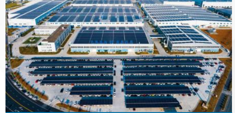
Ningguo, Anhui, China 15MW C&I Rooftop
