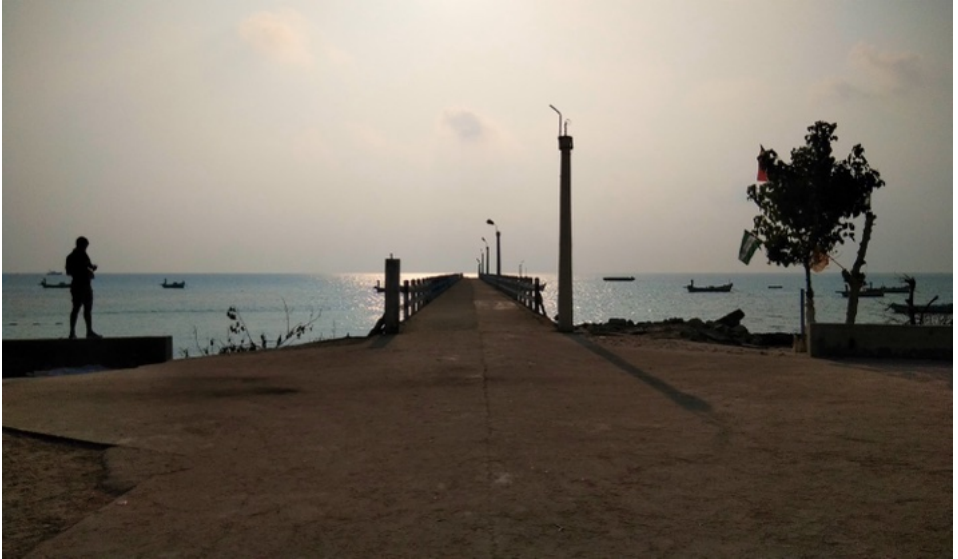
The Bitra jetty functions as the essential gateway to and from the island's massive lagoon. PHOTO BY SOMESH S. MENON
