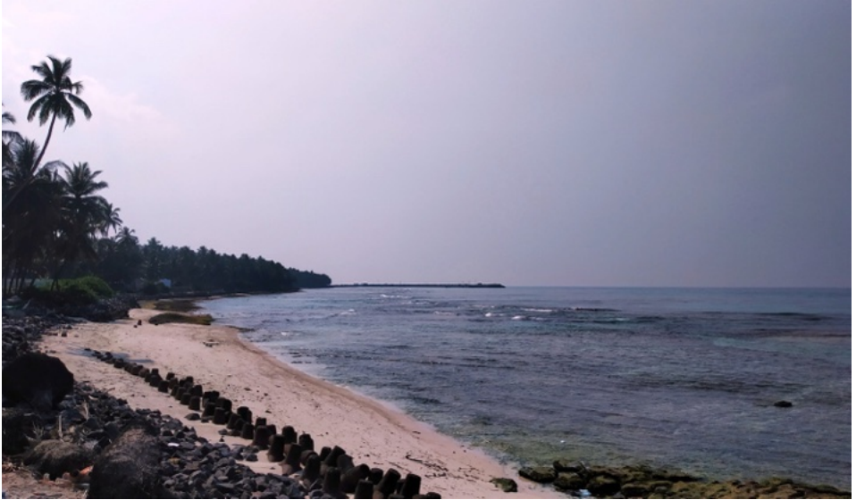
A distant view of Andrott's breakwater jetty, located on the northern side unlike other islands. PHOTO BY SOMESH S. MENON
