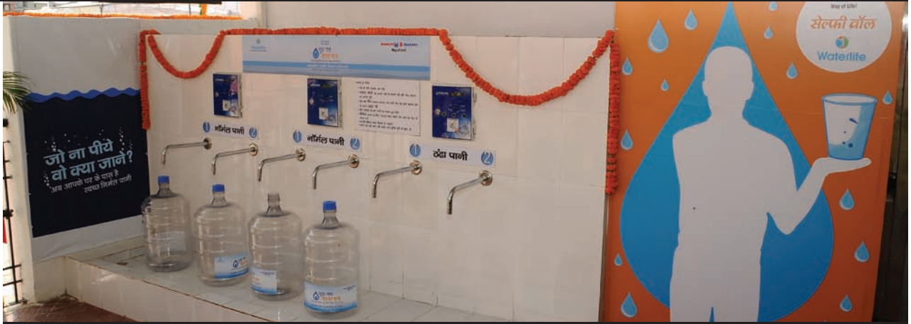
Water ATM - Community Safe drinking water project
