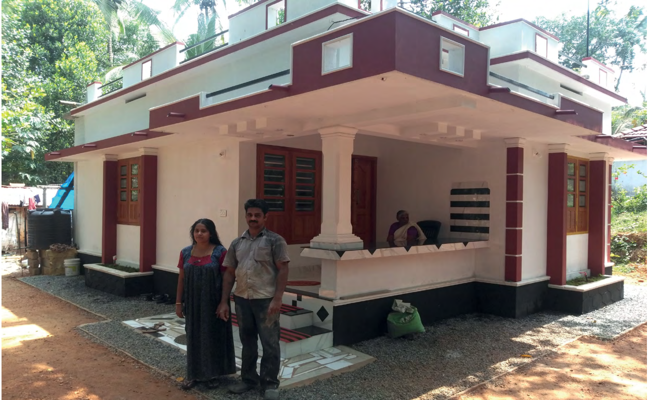
A house built under the Pradhan Mantri Awas Yojana-Urban in Goa. There is a demand for 11.2 million houses under the scheme in India
