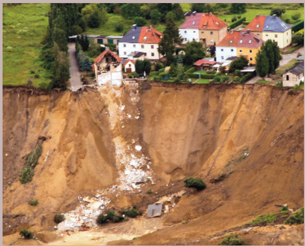
MINE BECOMES LAKE, SWALLOWS BUILDING A residential building and a road on the shoreline of a lake in a German village, Nachterstedt, collapsed on July 19. Three people are missing. Officials said the area had received some rain, but it is more likely that opencast coal mining in the past had made the land unstable. The lake was formed after the mine closed in 1991.
