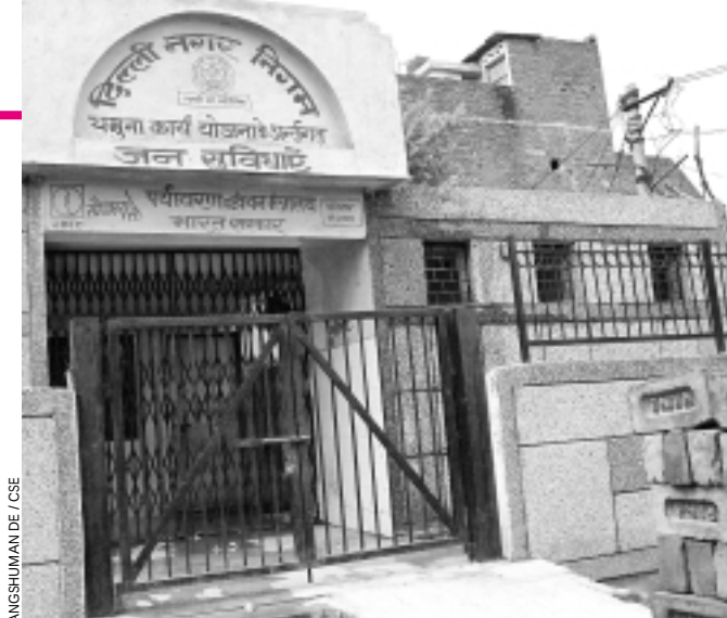
Going to waste: a YAP toilet lies locked
