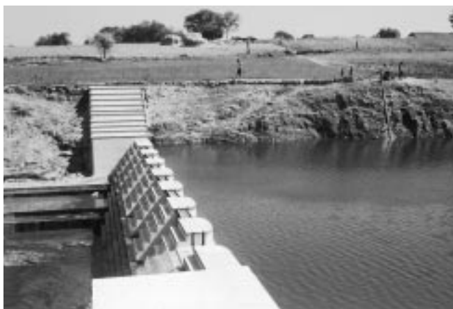
Structure of hope: a check dam built by the Sadguru foundation in Dahod, Gujarat, shows what the future depends on
