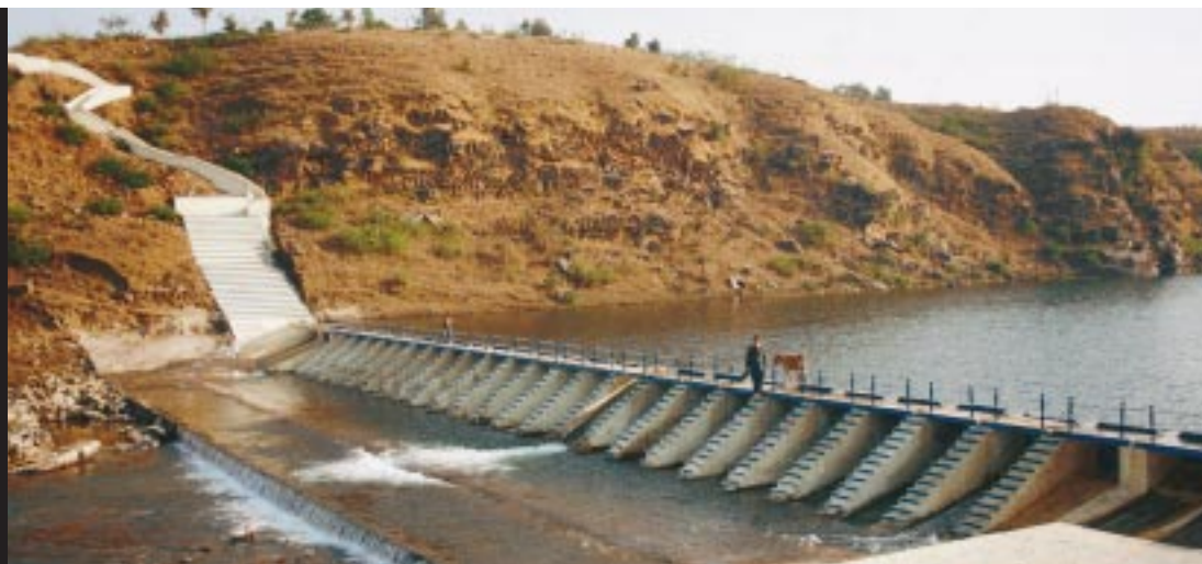
This check dam has captured more than enough water for irrigation till the next monsoon
