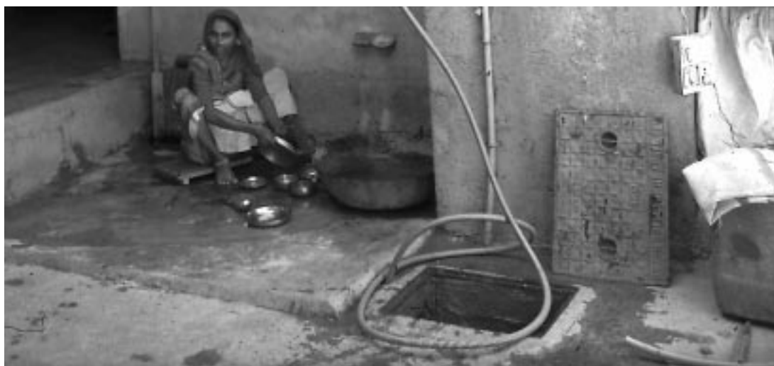
The water in the underground tank has been collected from the roof of this Mandlikpur house
