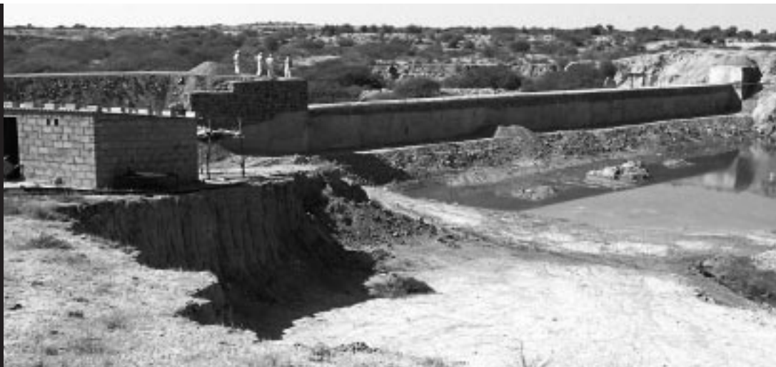
People of Gandhigram constructed this check dam with a bank loan and voluntary labour
