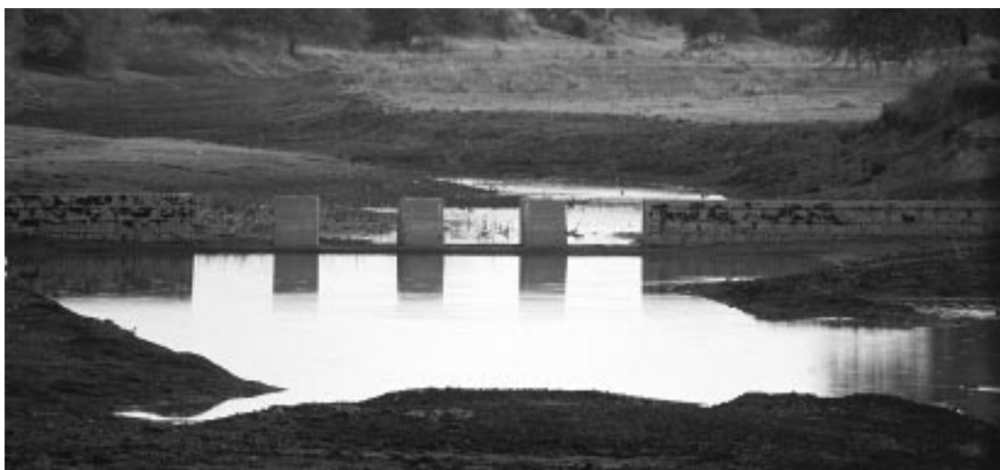
A check dam built at Raj-Samadhiyala village provides water for agriculture even during drought
