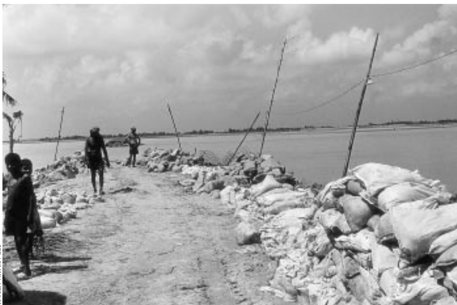
BAGGING CONTRACTS: Sandbags piled up by contractors as part of the relief and repair work being carried out on the spur of a retired embankment on Kosi
