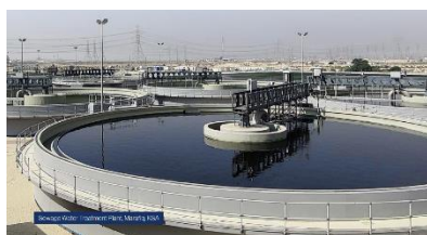
Sewage Water Treatment Plant, Marafiq, KSA
