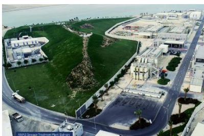
AMAS Sewage Treatment Plant, Bahrain
