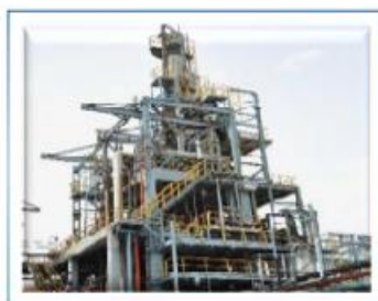
Chloromethanes plant, Mettur, Tamilnadu
